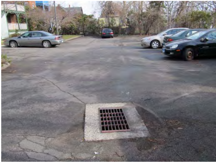
Original asphalt paving is in fair condition for its age
