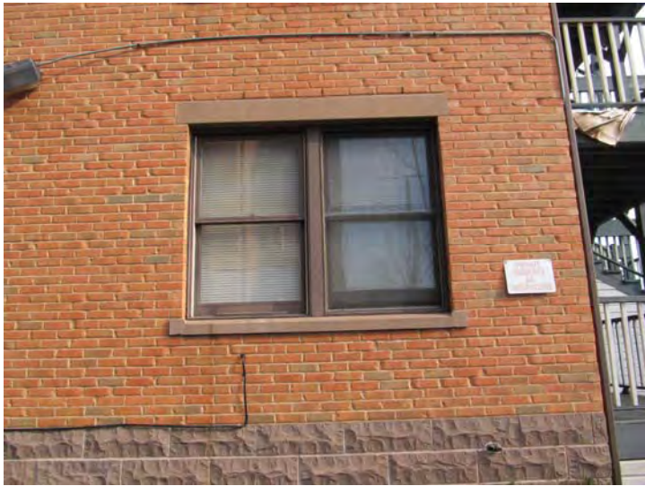
Typical original aluminum clad wood window assemblies – Note brick veneer is in good overall condition
