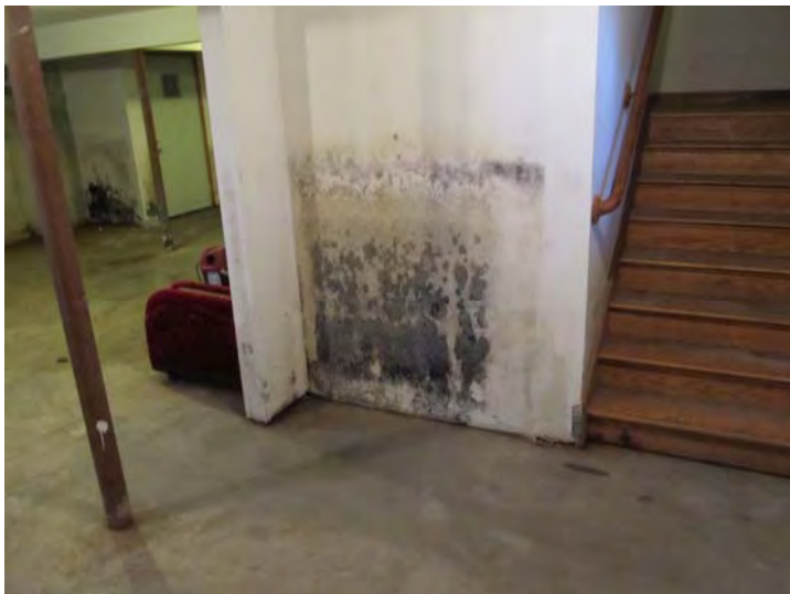
Recent flooding at basement level of #154 caused moisture damage to drywall surfaces – Repairs and new sump pump installation to occur in spring of 2013
