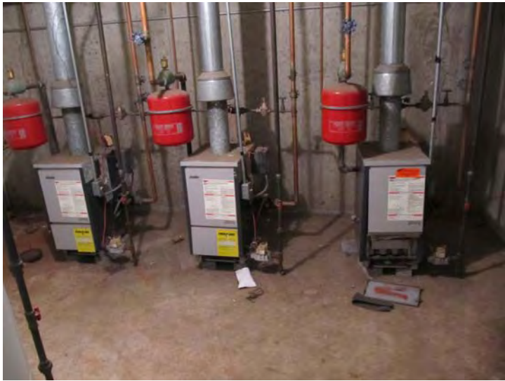
Each unit has its own natural gas-fired boiler for production of hydronic heat – Boilers are original and nearing the end of their expected useful lives
