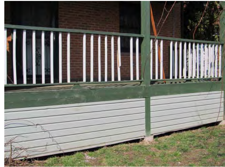
Typical condition of railings and porches – Selective repairs needed at various locations
