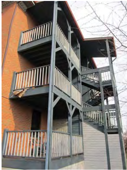
Typical multi-story wood-framed rear porch/egress system at each building
