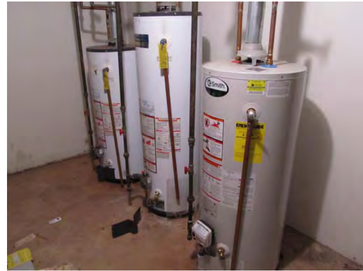
Individual natural gas-fired tanks of varying ages and brands of manufacture serve unit-level domestic hot water needs
