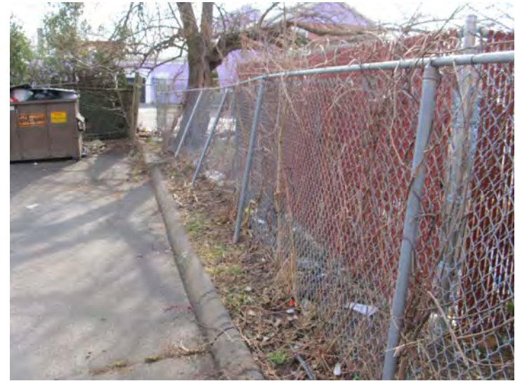
Damaged chain link fencing along side of parking area – Damage the likely result of snow removal operations
